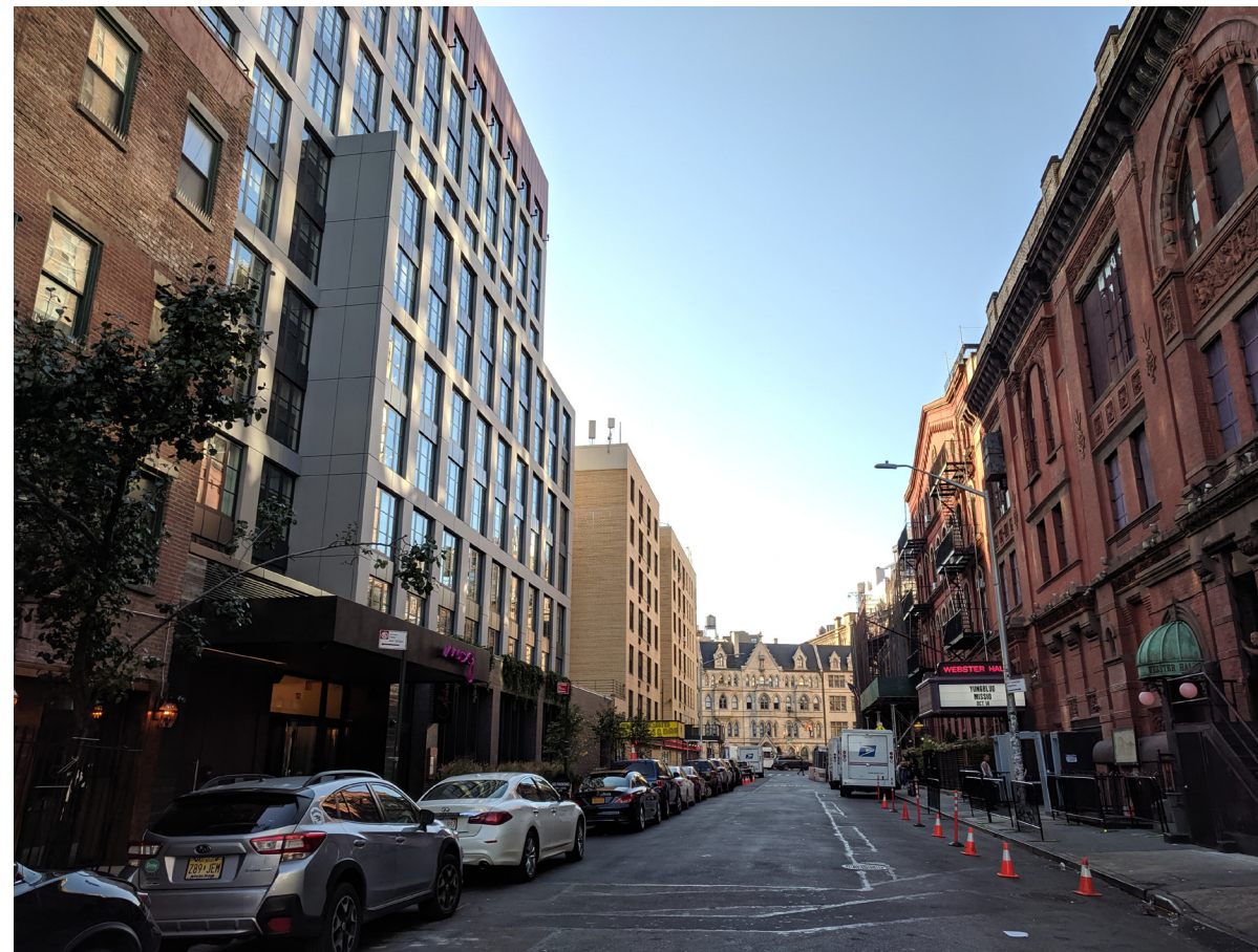
32. East 11th Street looking west - Moxy Hotel & Webster Hall
