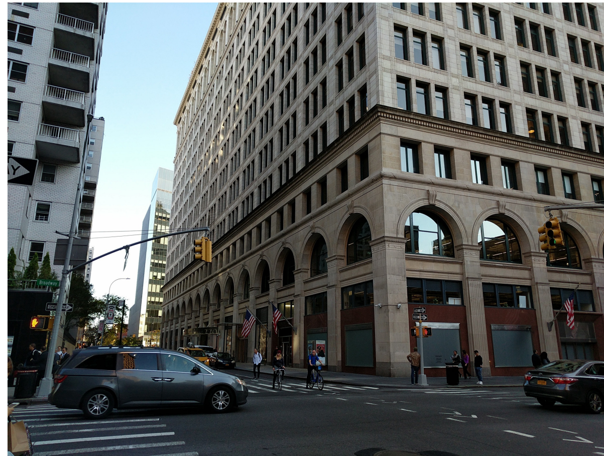
28. Broadway and East 9th Street looking southeast
