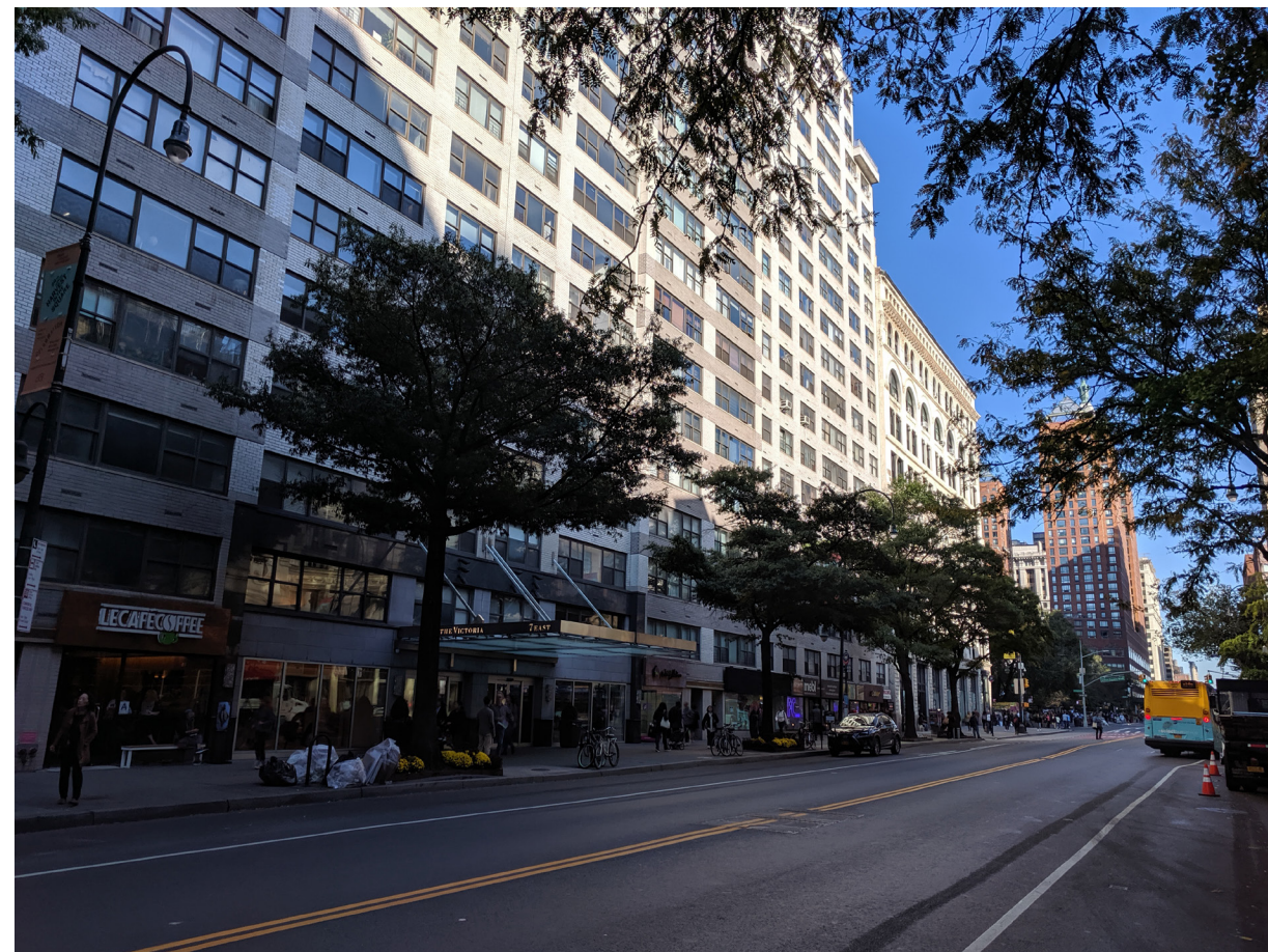
4. 14th Street looking northeast
